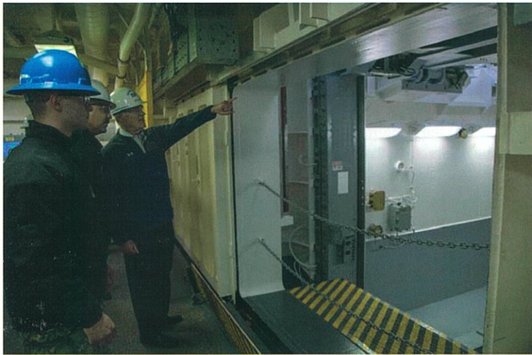
ECNAV is briefed by CVN-78 OHO on US-1 Advanced Weapons Elevator
