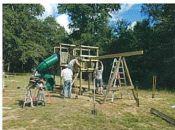
Putting up and fixing some rotten boards on the playground
